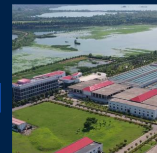
Huaihe River Water Diversion Project
