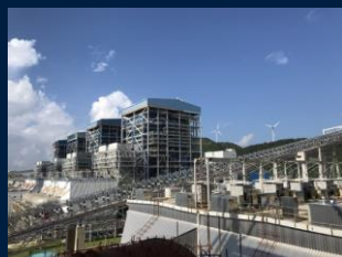
Huaxia Yangxi Environmental Protection Island Project, the largest one in China in terms of total installed capacity
