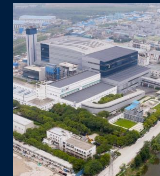
Shanghai Electric Nantong Waste Incineration Cogeneration Project
